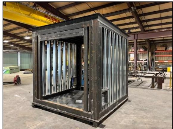
Fabrication of our storage building, as of March 5th
